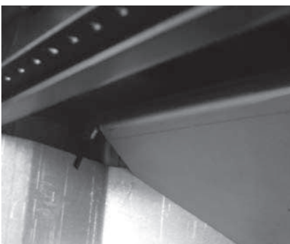
Pict. 15: Lift the fire shield
